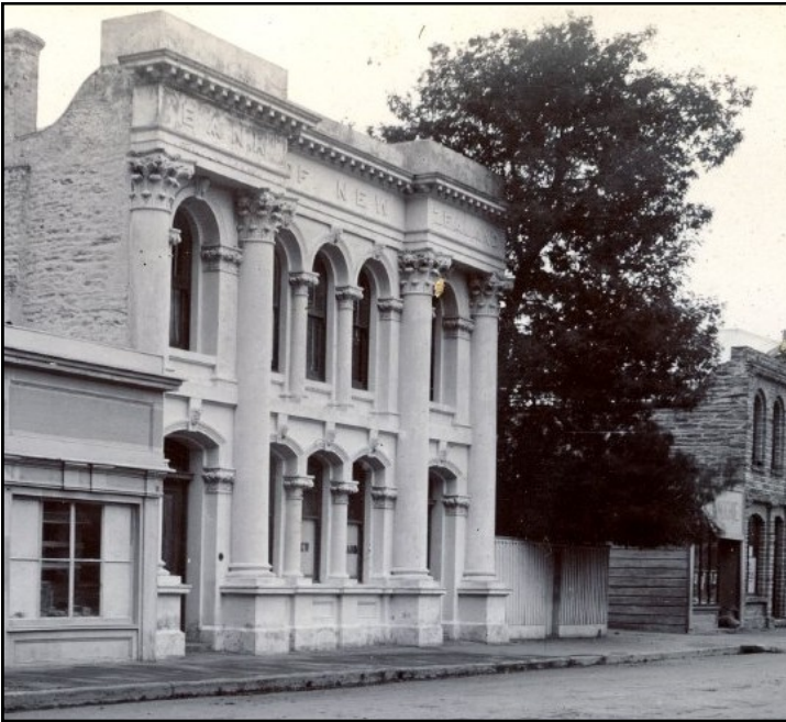
Bank of New Zealand, Rees St, Queenstown built in 1875, seen here not long before demolition. (LDM EL1602)
